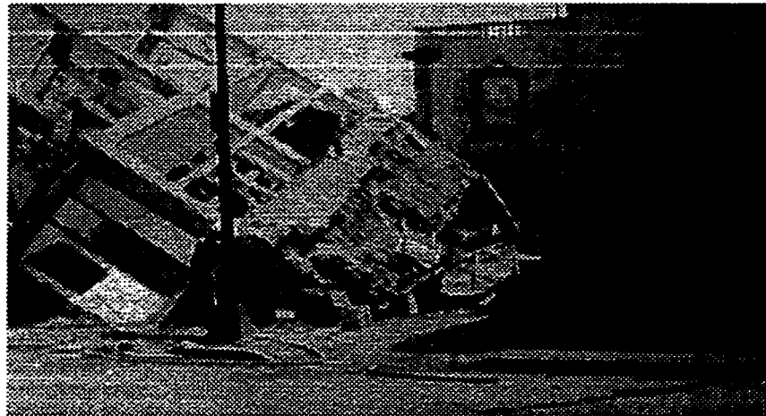
Figure 8.2 Structural Collapse Due to Soil Liquefaction
