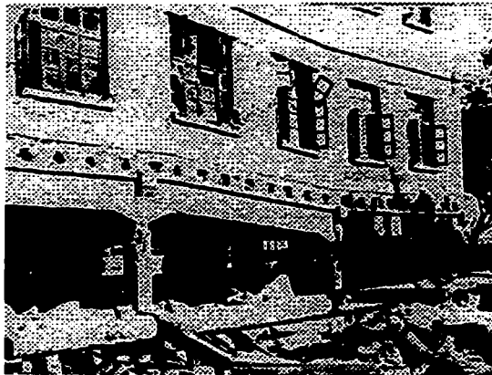
Figure 2.8c Stiffness Discontinuity
