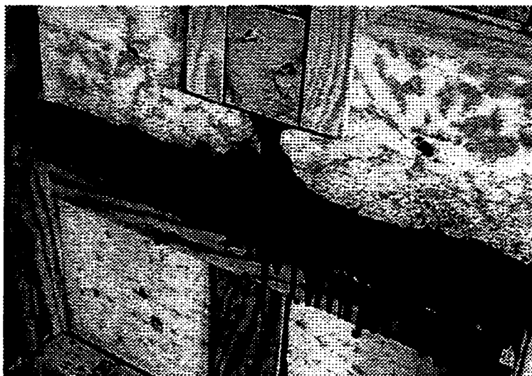
Figure 3.12a Trough Method of Strip Grouting
